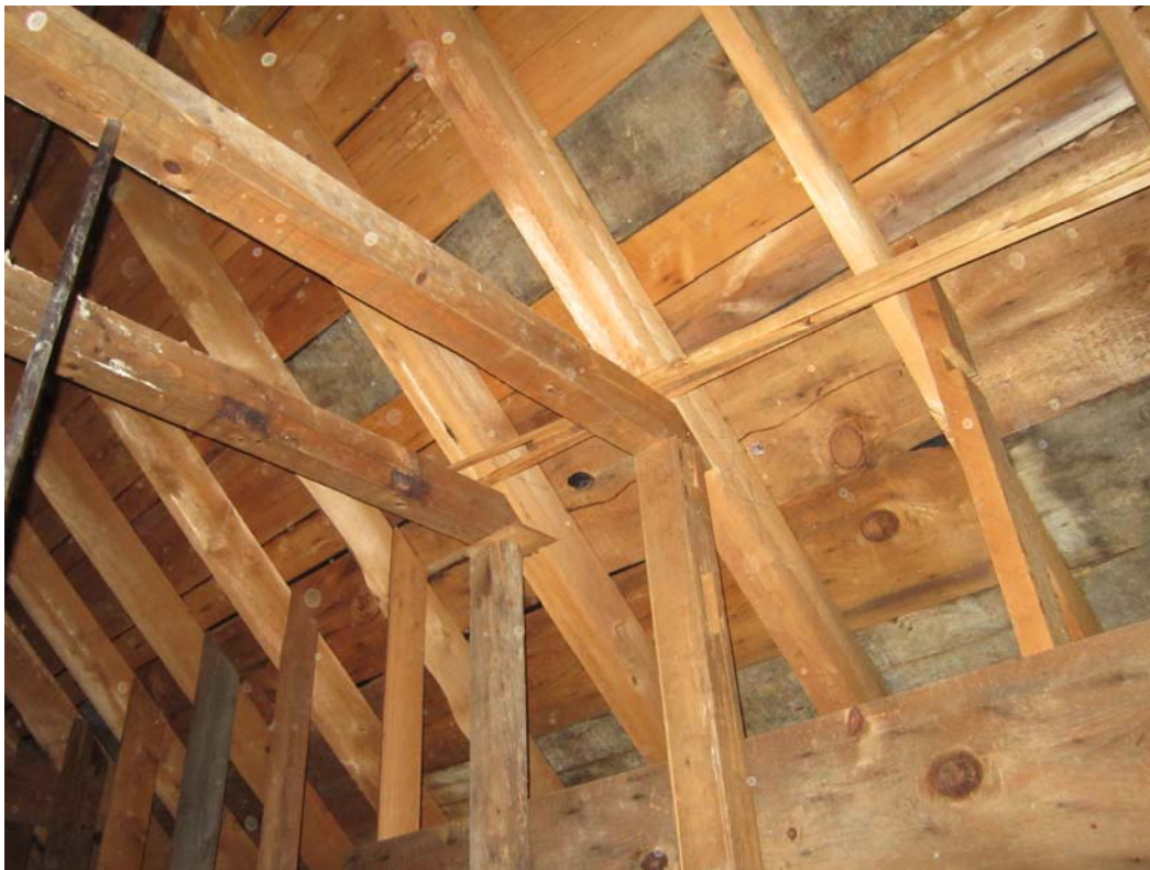
Attic with sawn common rafters. Additional framing to left was apparently added for lateral support of recently removed hanging chimney at center of meeting hall.
