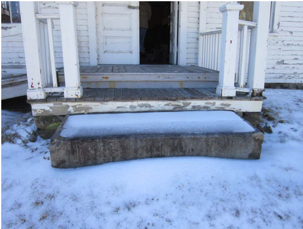
Porch floor is in very poor condition related to trapped moisture in the current assembly
