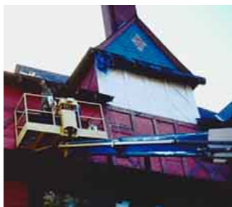
A heat plate was used on the cornice to remove paint. Photo: NPS files.
