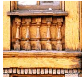
When the protective and decorative paint finish was removed and an inappropriate clear finish applied, the exterior character of the building was altered. Photo: NPS files.
