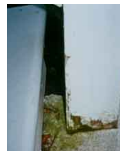
The problem evidenced here by mossy growth and deteriorated wood must be resolved and the wood allowed to dry out before the wood is repainted. Photo: NPS files.
