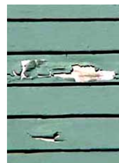
Peeling paint on historic wood siding. Photo: ©John Leeke, 2002.
