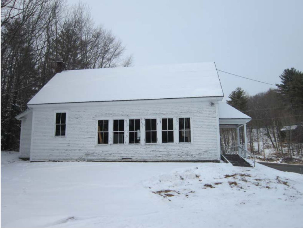
South elevation of main block with the privy seen to the left and the entry porch on the right side with its overlaid non-conforming ramp.
