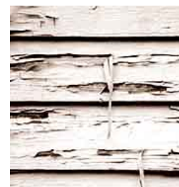
Extensively deteriorated paint needs to be removed to bare wood, then primed and re-painted. Photo: NPS files.
