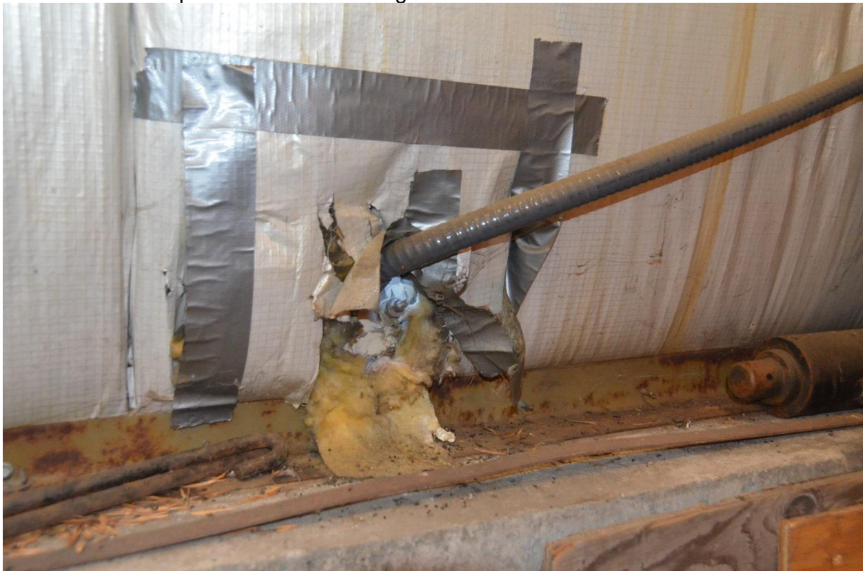
Above: Poor seal (but in unheated portion).
