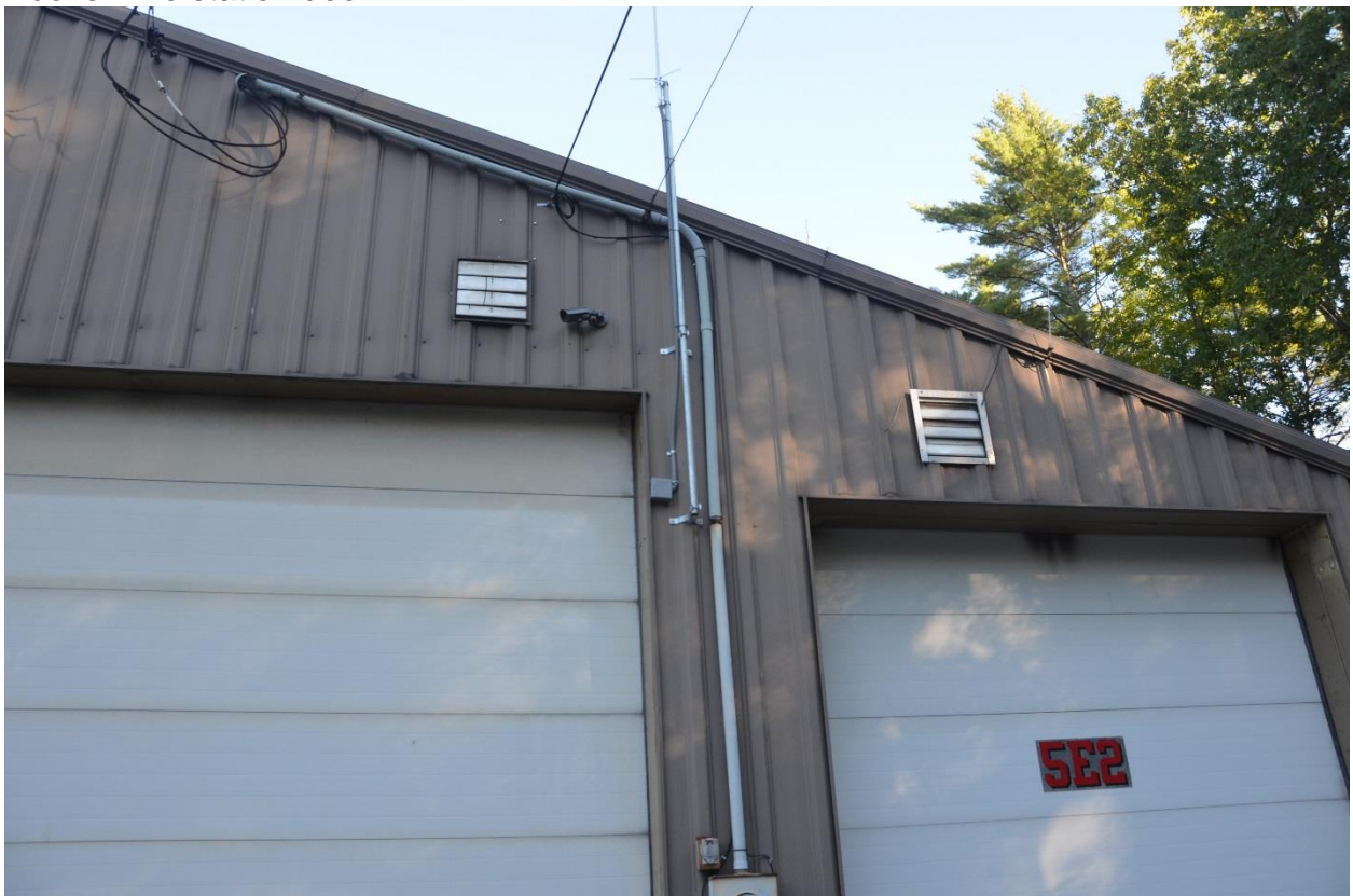
Above: Louvered fans may need to be replaced? Weather stripping on doors is not in good shape.
